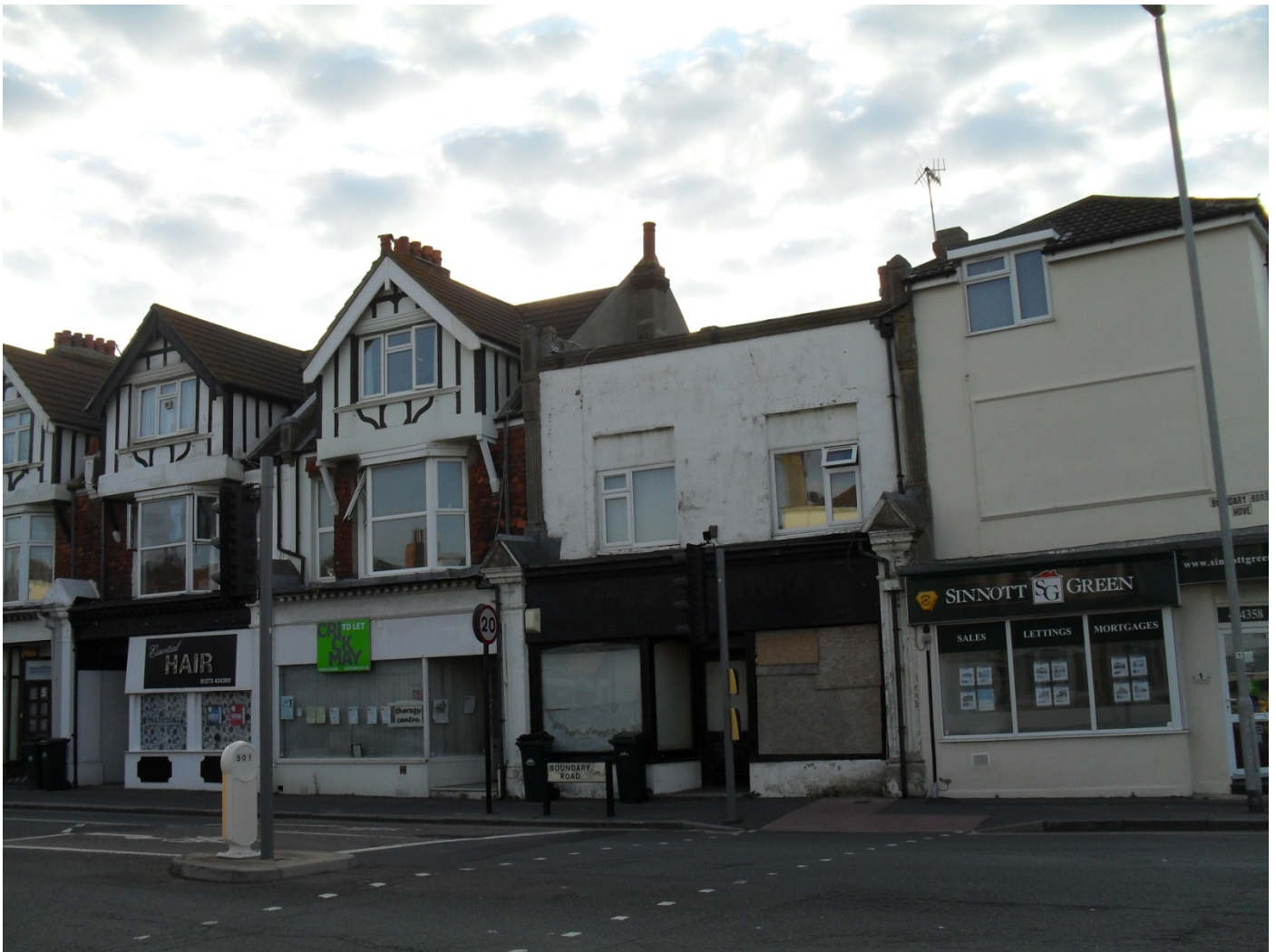
FIGURE 1 NUMBERS 4,3,2,1 BOUNDARY RD – NO 3 HAS A GREEN SIGN BOARD
